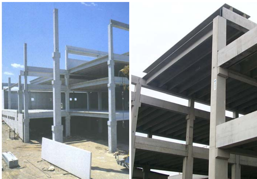
Figure 1. Precast multi-storey frame structures during erection.
