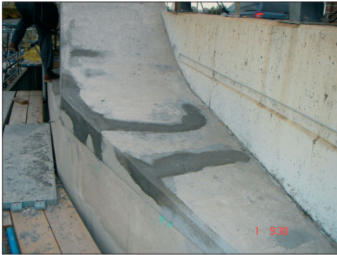
(c) Local sutures with tixotropic, anti-shrinkage, polypropylene fiber reinforced mortar
