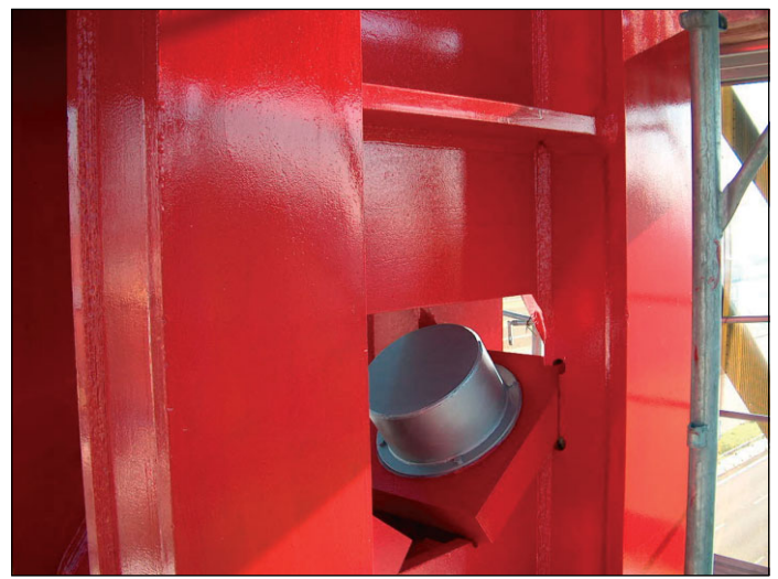
(b) Detail of the anchorage assembly after painting
