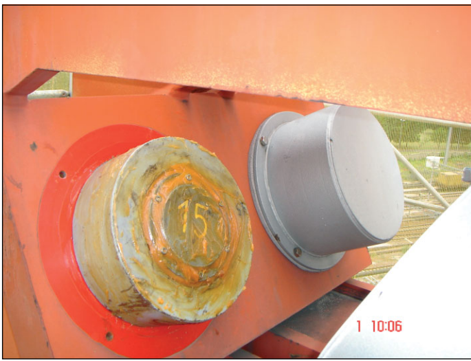
(a) Head of the anchorage cable inspection
