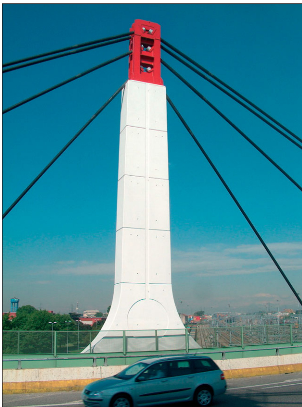
Fig. 7: View of a pylon after the rehabilitation intervention
