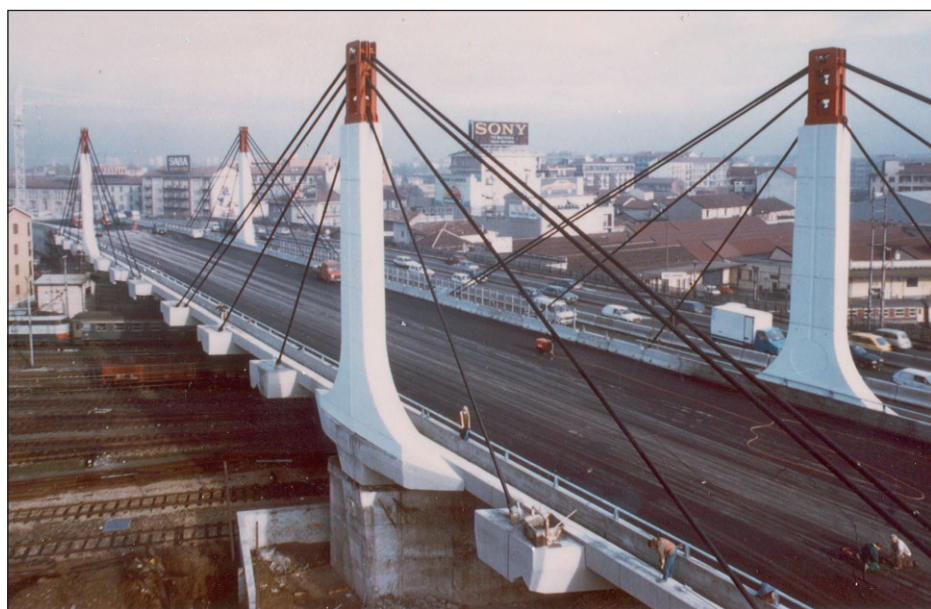
Fig. 1: View of the Certosa cable-stayed bridge
