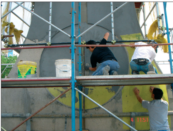
(e) Skin protection with high adhesion elasticity sealing cement mortar, reinforced with double or simple skin mesh
