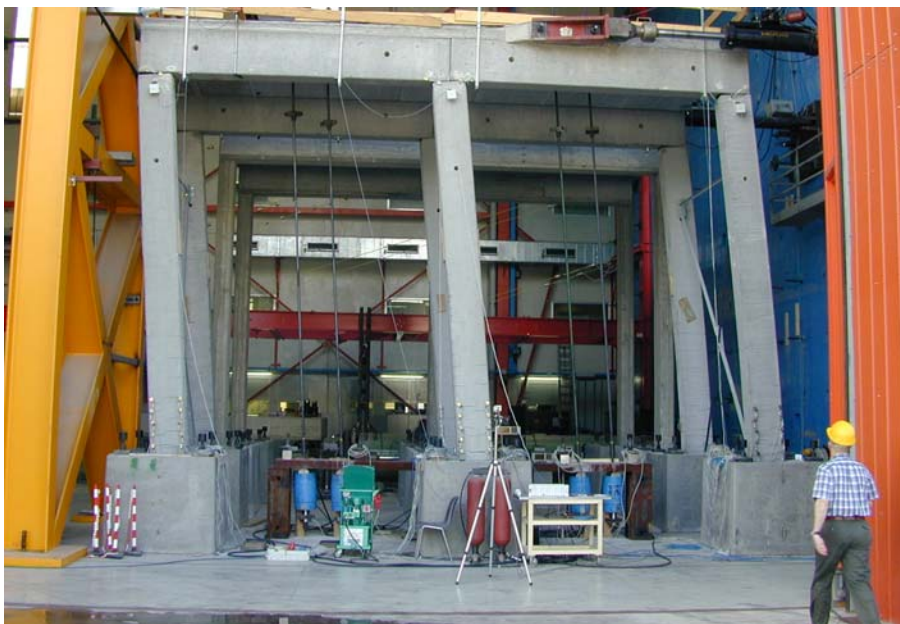
Fig. 16. View of the precast prototype at the end of the pseudodynamic test.
